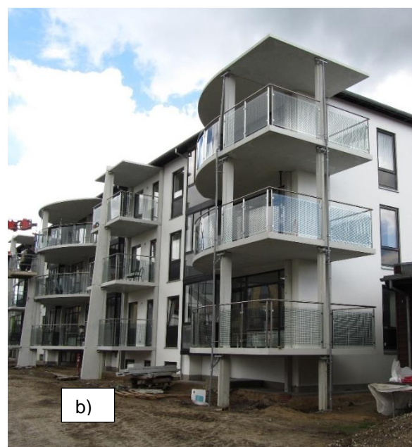
Figure 2: Cantilevered balcony element placed on corbels in the bottom of the deck and with bolted connections transferring tensile forces into the façade from the top of the balcony upstands.
