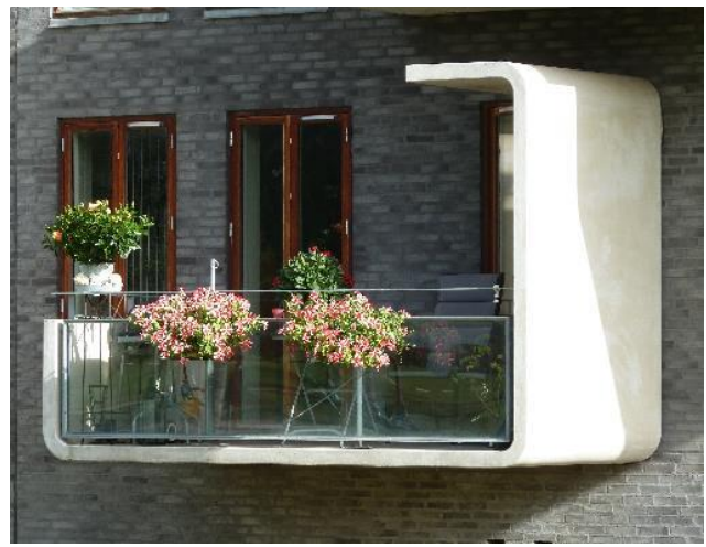
Figure 2: Cantilevered balcony element placed on corbels in the bottom of the deck and with bolted connections transferring tensile forces into the façade from the top of the balcony upstands.
