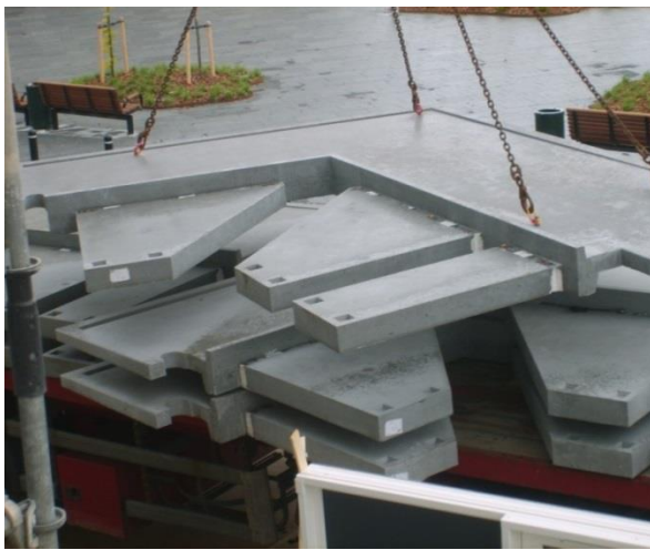
Figure 1: Cantilevered balcony elements ready for installation. The cantilevered flaps are cast monolithically as part of the element for attachment to the building floor.
