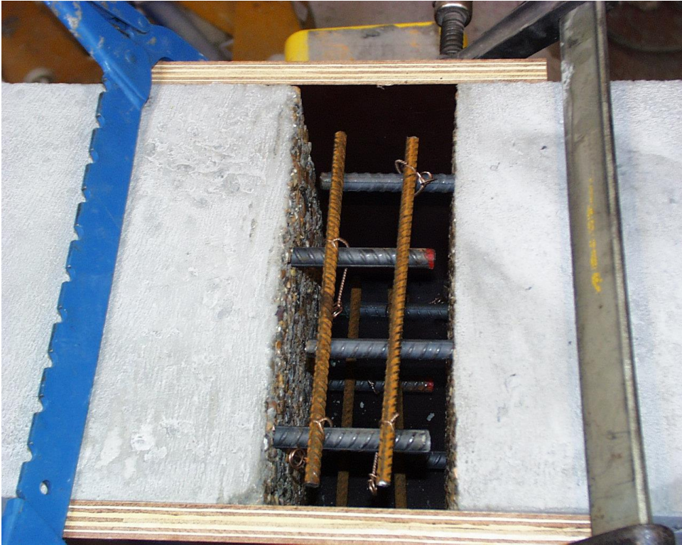
Figure 7: Beam specimen with lapped \varnothing 12 mm bars before casting.
