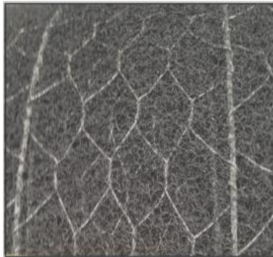
Figure 5 - Double twisted wire mesh reinforced with ropes and with additional geomat
