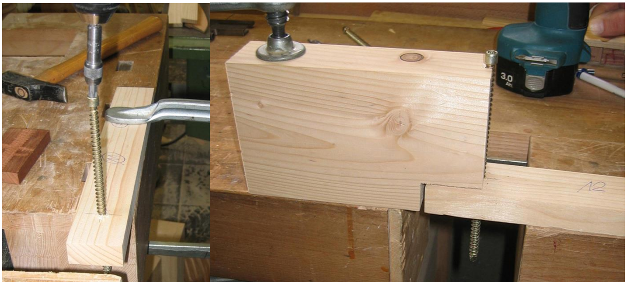
Fig. 1: Inserting a screw using a template made of timber.
