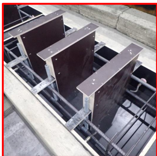
Figure A.1.2.1.3: Example for additional formwork panels
