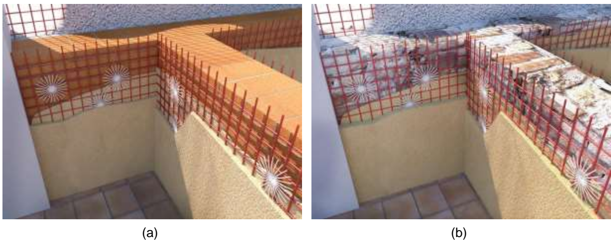
Figure 1.1.3: Kit for strengthening of masonry and reinforced concrete: (a) application on clay masonry; (b) application on natural stone masonry
