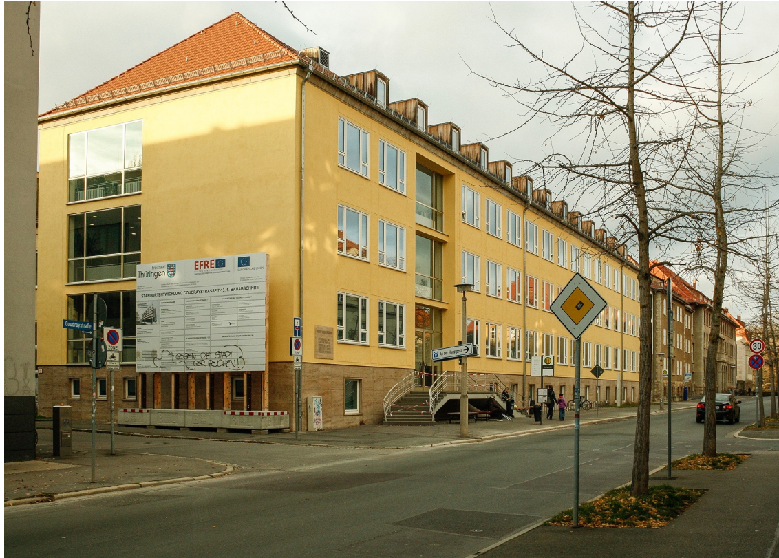
Energy-oriented refurbishment of a historic building with a high-performance aerogel insulation plaster covered by ETA-20/0277 based on EAD 0415559-00-1201
