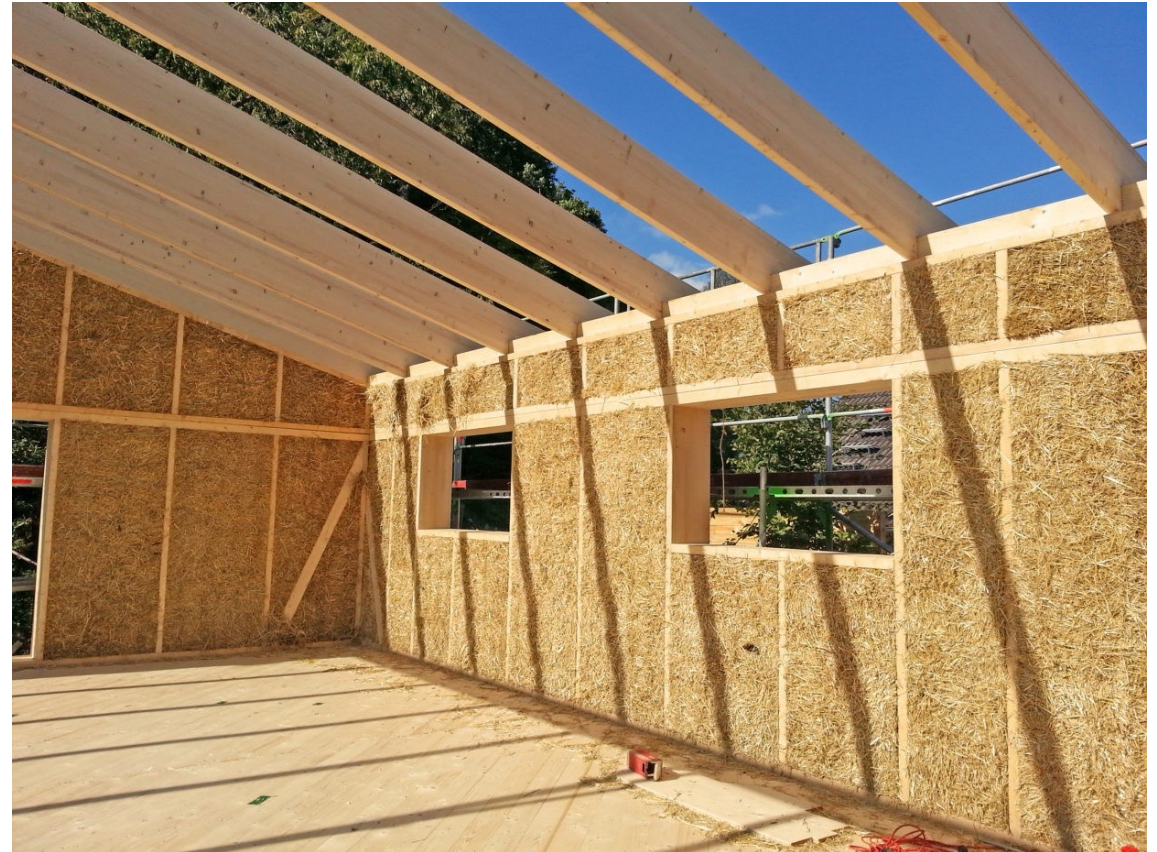
Thermal insulation made of straw (ETA-17/0247 based on EAD 040146-00-1201) Source: FASBA e.V., Verden (Aller)
