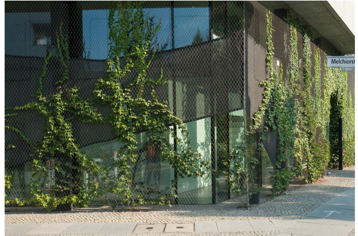
ETA-assessed cable net systems for green facades Source: DIBt
