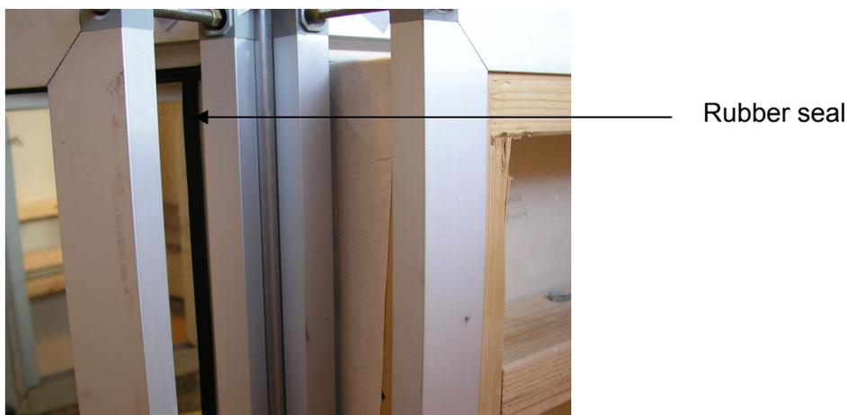
*Figure 2. Sealing with a soft (hollow) rubber profile.*
